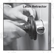
Insert the Lock Motor so that the latch retractor faces the edge of the door.
