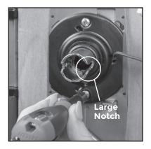
Align the Inside Lever Post so the large notch faces away from the edge of the door. Attach the Inside Lever Post to the Mounting Plate using two (2) M6x10mm screws.
